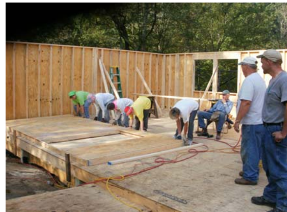
New House Walls being Raised
