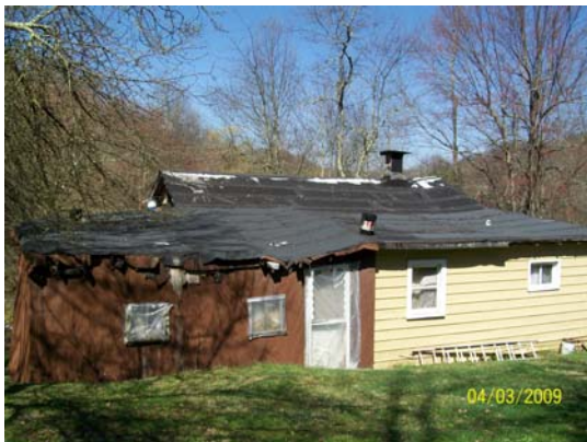
Emma's Old Home (before demolition)
